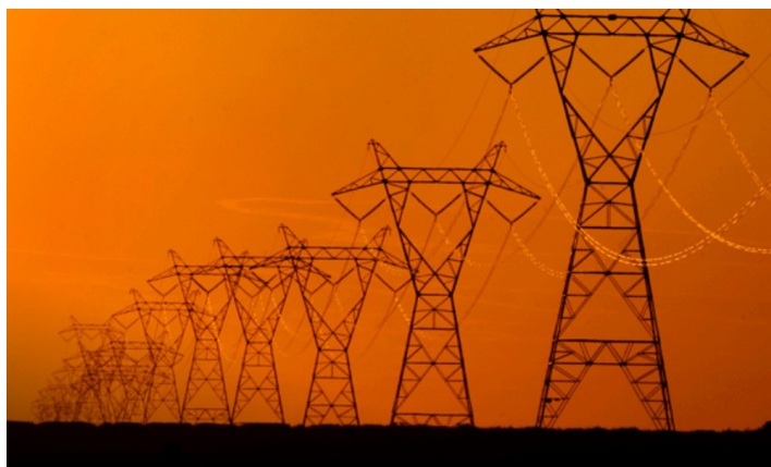
Figure 1: Using transformers, utilities can transmit power thousands of kilometers
