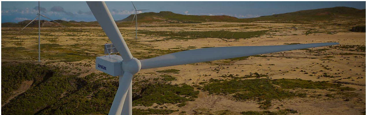
Figure 11: Vestas V172-7.2MW wind turbines
